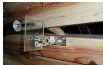
a) Large deformation of dowel
