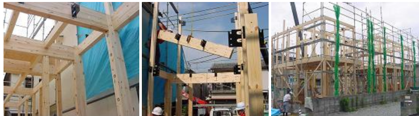
Figure 1. Typical construction site of modern wooden post and beam style residential house.
